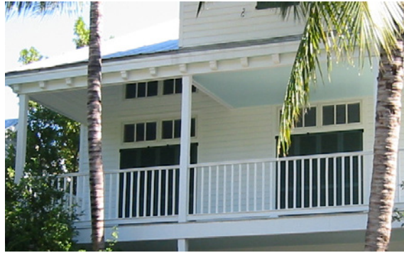
Typical porch construction
