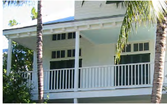
Typical porch construction
